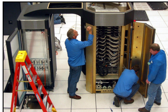
Figure 1. Cray technicians installing a portion of the AHPCRC's liquid-cooled X1 system at NetworkCS, Inc. (Minneapolis, MN) on February 20, 2003.
