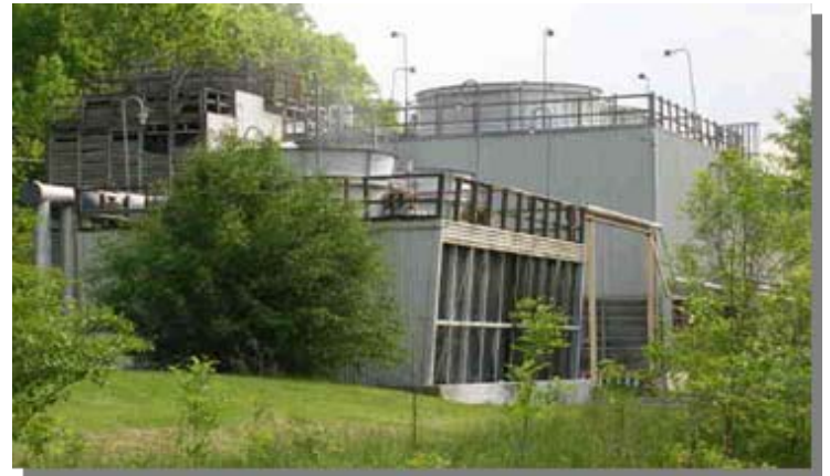
30+ MW Central Chiller Plant
