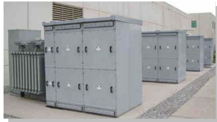
13,800 volt transformers for computers and infrastructure
