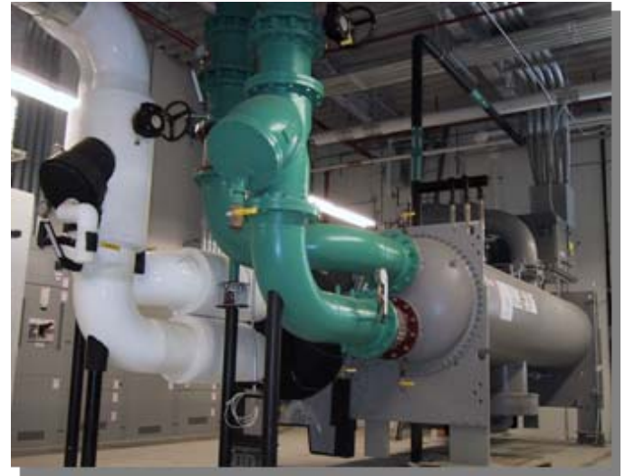
Cooling today for 8 MW with hot-spare
