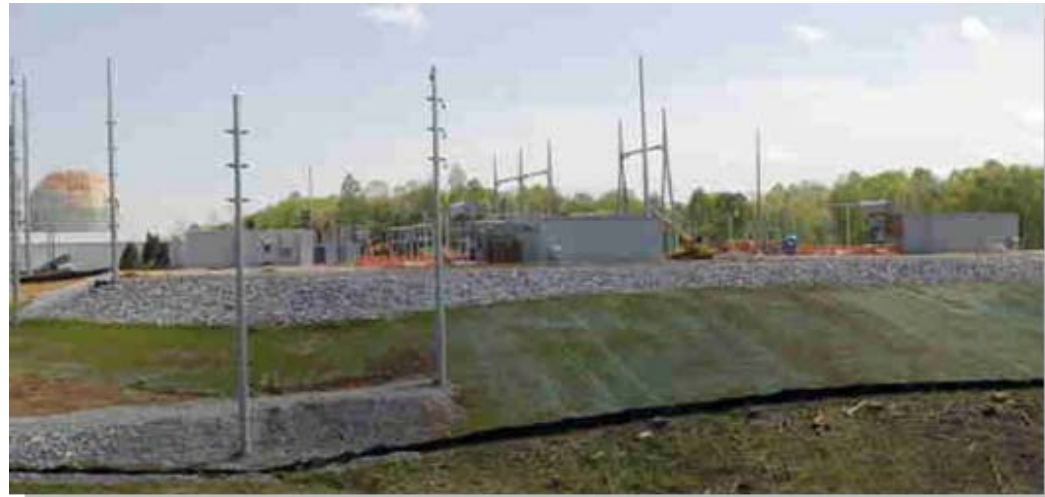
New Power Substation Under Construction
