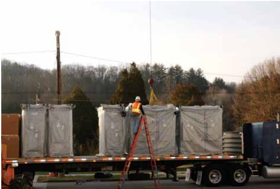
Distribution equipment arrives as part of the 15MW expansion of electrical capacity.
