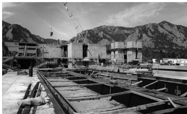
Figure 1. The National Center for Atmospheric Research, under construction in 1965.
