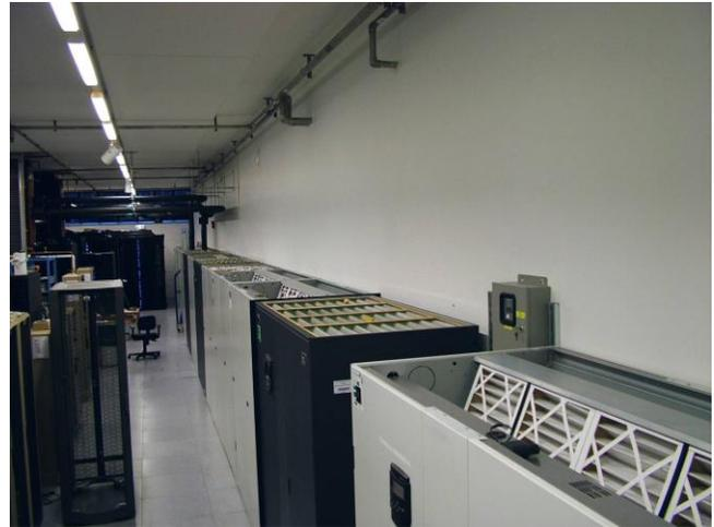
Figure 3. Row of computer room air conditioners (CRACs) in the PDC computer hall.
