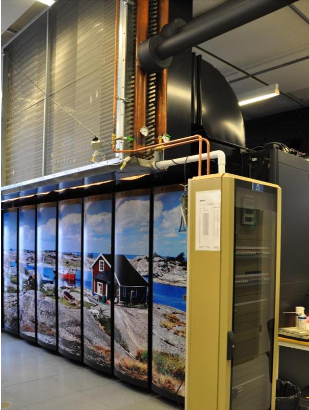
Figure 5. Custom made ducts on top of the Cray lead the air through industrial heat exchangers.
