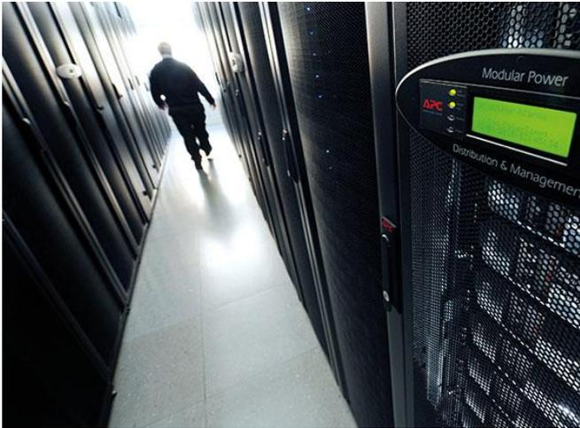
Figure 2. Encapsulated hot aisle in the APC cooling.
