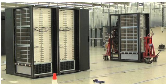
Figure 2: Placing the XC30 cabinets using the wheeled lifting equipment.
