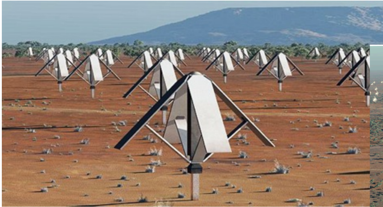
SKA Phase 1 Low Frequency: 900 Station x 300 Antennas/Station
