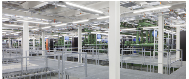
Figure 1. Image of the Installation Deck showing the supporting I-beam structure, PDUs and system-dedicated cooling loops.
