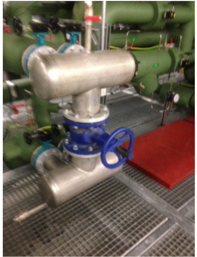
Figure 5. Photograph showing the pipework, prior to lagging, for one of the primary- to secondary-side heat exchanger by-passes, including cross-connect valve.
