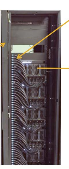
Tubes move cooling liquid to and from RackCDU to servers.
